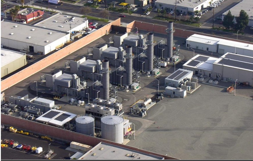
Figure 2. Canyon Power Plant
