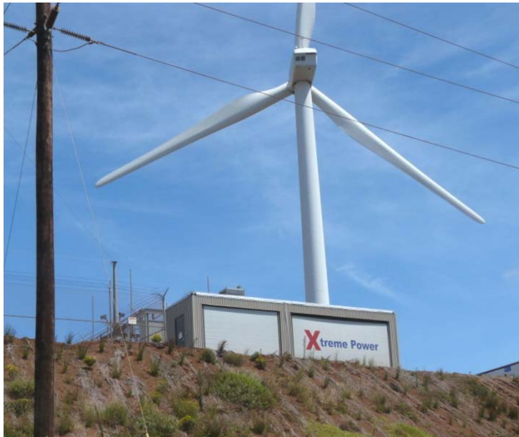
Figure 3.5 1.5-MW/1-MWh Advanced Lead-acid Dry Cell Systems by Xtreme Power in a Maui Wind Farm
