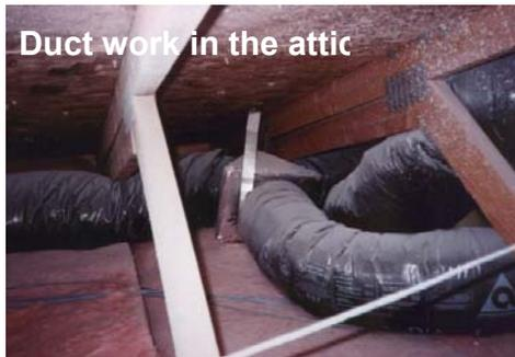
When ducts are located in a hot attic, the cool air inside them warms up before it reaches the rooms you want to air condition. Air leaks are also inevitable. When cool air leaks from a duct into a hot attic, more energy and money are expended to keep a home comfortable.
