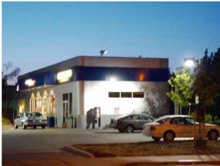
Source: AEC. Photographer: Tom Bergstrom
