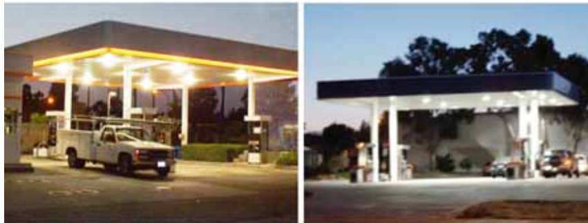
Source: AEC. Photographer: Tom Bergstrom
