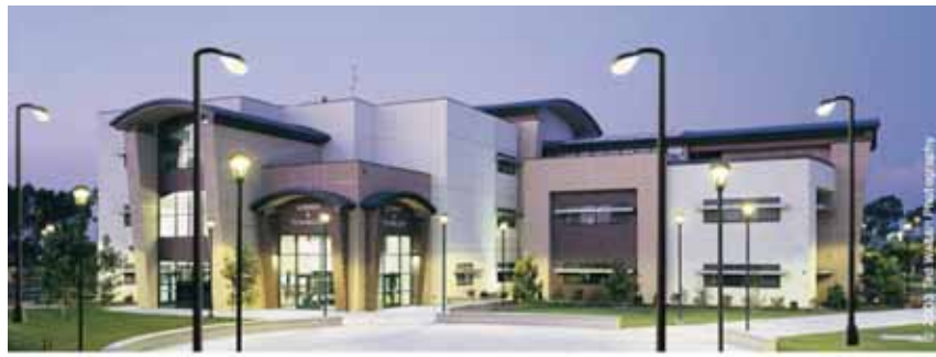
Figure 6-9– Ornamental Lighting (The cobra head luminaires shown in the above figure are not ornamental lighting. However, if the post-top acorn luminaires are rated 100 watts or less, they qualify as ornamental lighting)
