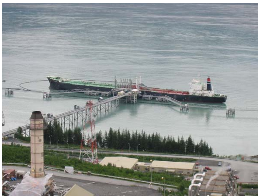
Figure 3: Marine Terminal Facility
