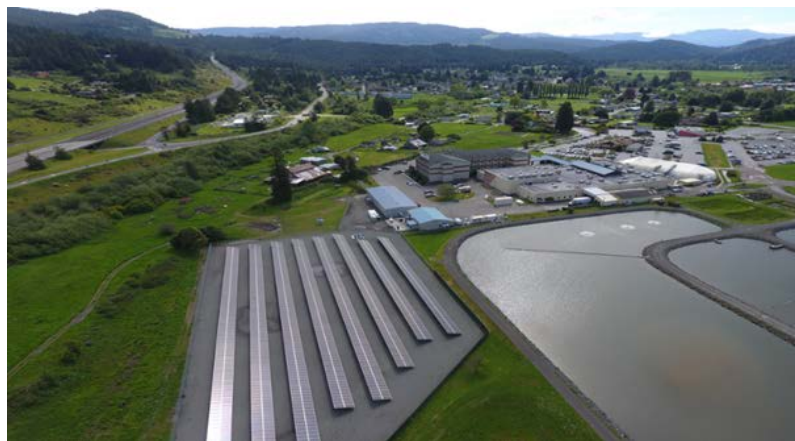
Figure 2: Blue Lake Rancheria Microgrid
