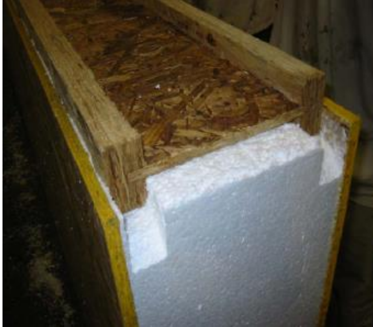
Figure 13: Insulated Manufactured Home Envelope Component
