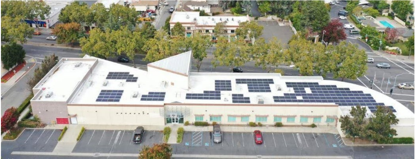
Figure 3: Aerial View of Demonstration Site
