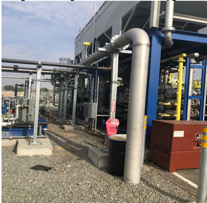
Figure 11: Biogas Connection to the Upgrader
