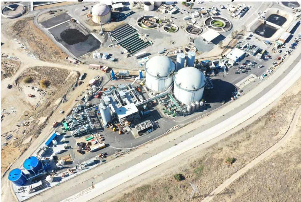
Figure 1: Rialto Bioenergy Facility
