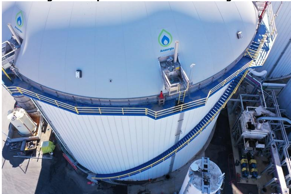
Figure 2: Top View of the Anaerobic Digester
