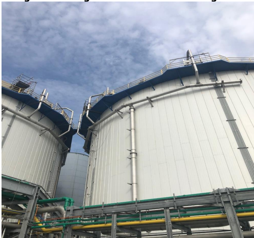
Figure 19: Biogas outlet to Anaerobic Digester
