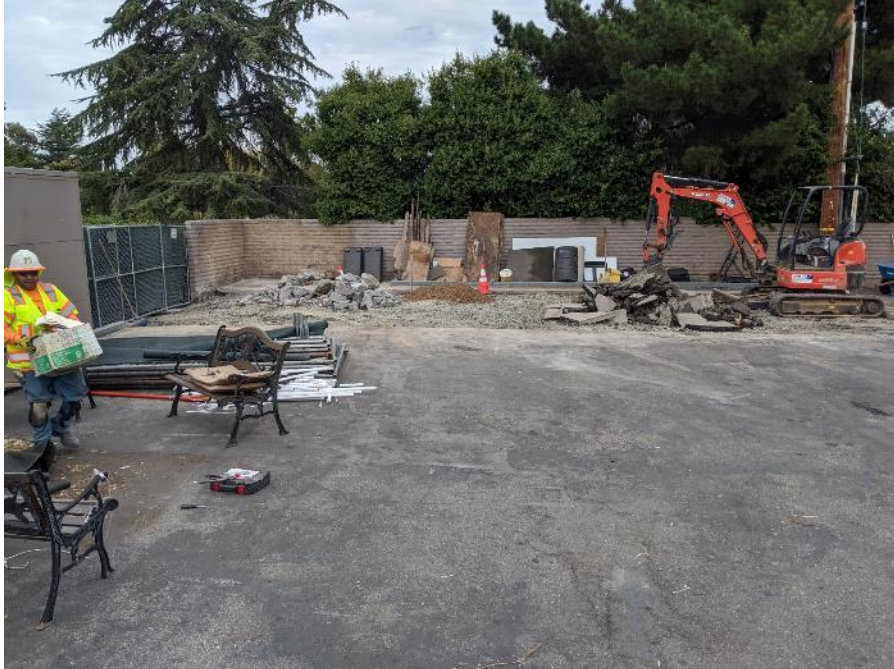
Figure 6: Breaking Ground at the Campbell East Hamilton Station
