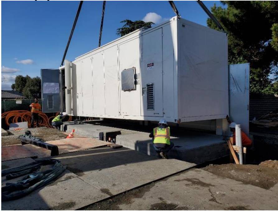
Figure 7: Linde Equipment Installation at the Campbell East Hamilton Station
