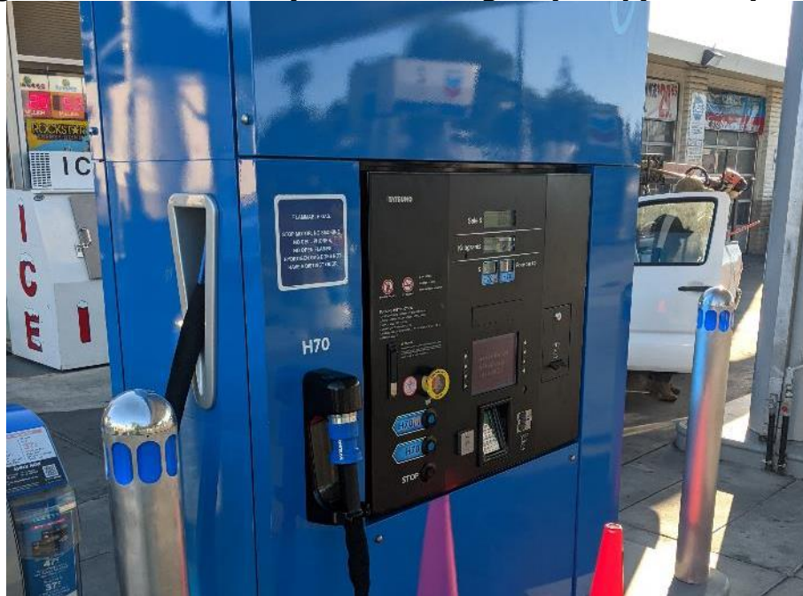
Figure 9: DMS Sticker (next to Emergency Stop) on Dispenser
