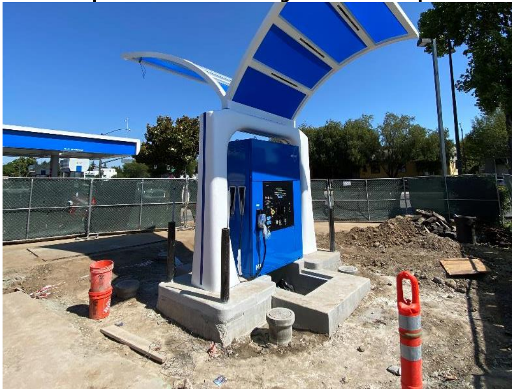
Figure 8: Tatsuno Dispenser Installation Progress at the Campbell Hamilton Station
