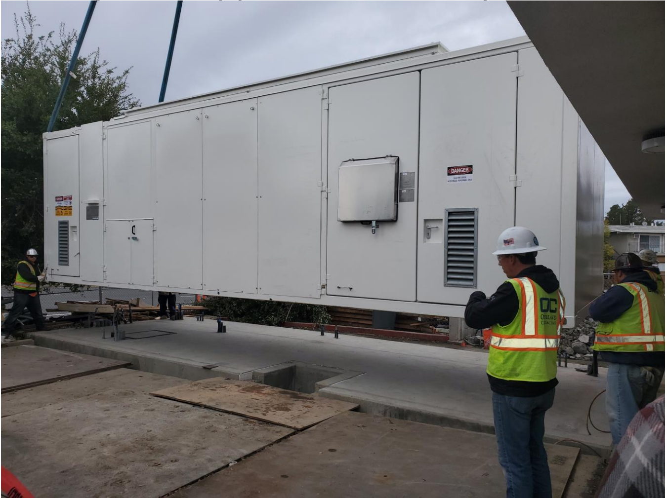
Figure 7: Linde Equipment Installation at the Sunnyvale Station
