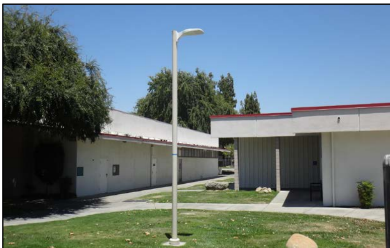
Photo Caption: New LED lighting at Porterville College in Porterville, CA Source: California Community College Chancellor's Office
