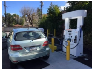
Photo Credit: Air Products and Chemicals, Inc.
