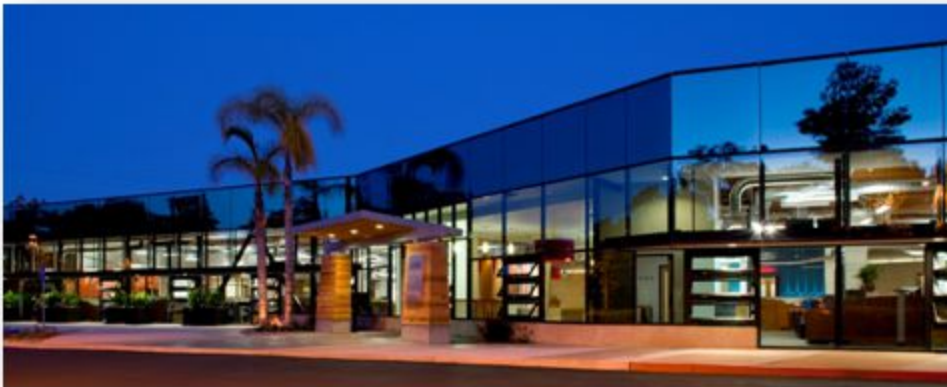
DPR Construction San Diego Corporate Office , Chip Fox, DG&E, renovation
