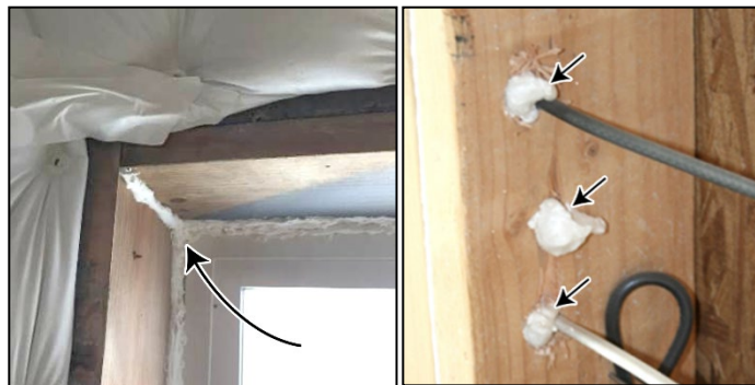
Figure 3-10: Air Sealing
