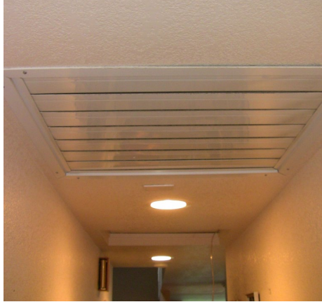
Figure 4-38: Whole-House Fan With Barometric Damper
