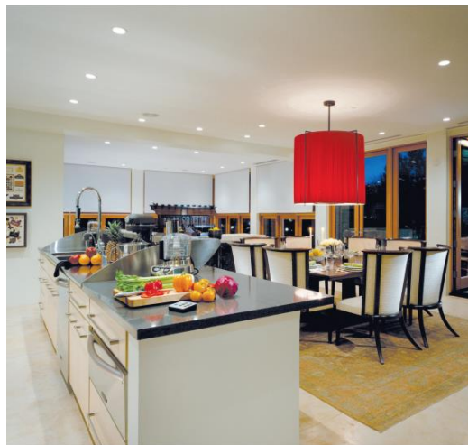
Figure 6-1 Recessed Downlight Luminaires in Ceiling
