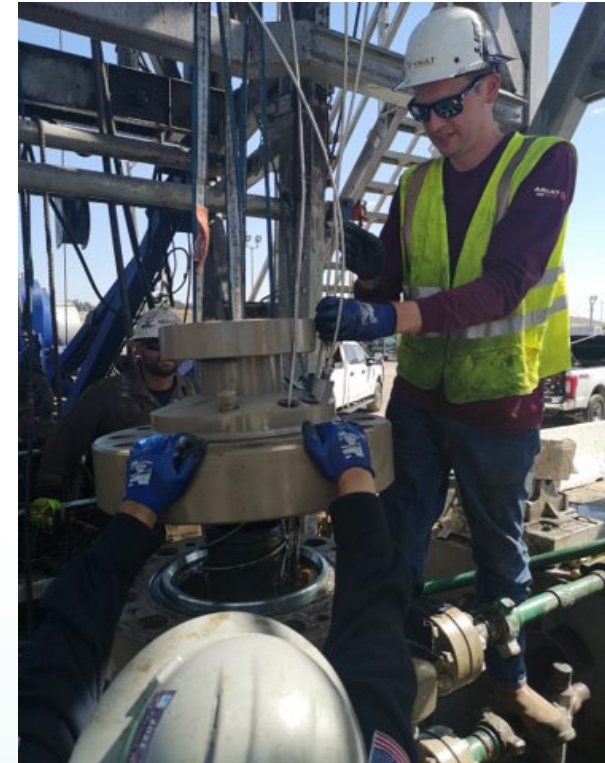
Fiber Optics Installation at PG&E's McDonald Island Gas Storage Field Source: LBNL
