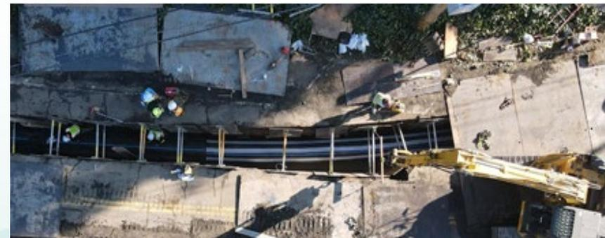
DFOS installation on water pipeline near Hayward fault; Source: UC Berkeley
