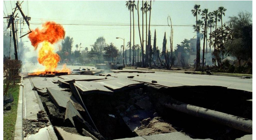
Failure and explosion of gas pipeline, Balboa Blvd, Northridge, 1994; Source: LA Times
