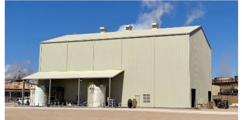
BHE Renewables \text{LiCl}^2 demonstration plant in operation since June 2022
