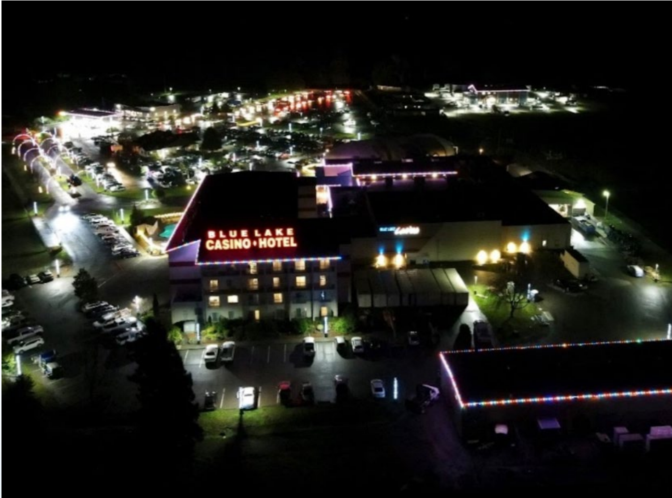
Photograph of Blue Lake Rancheria, Source: Schatz Energy Research Center
