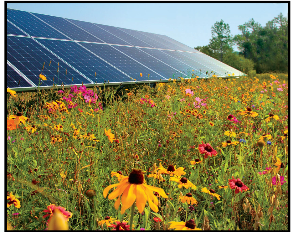
Source: Encore Renewable Energy
