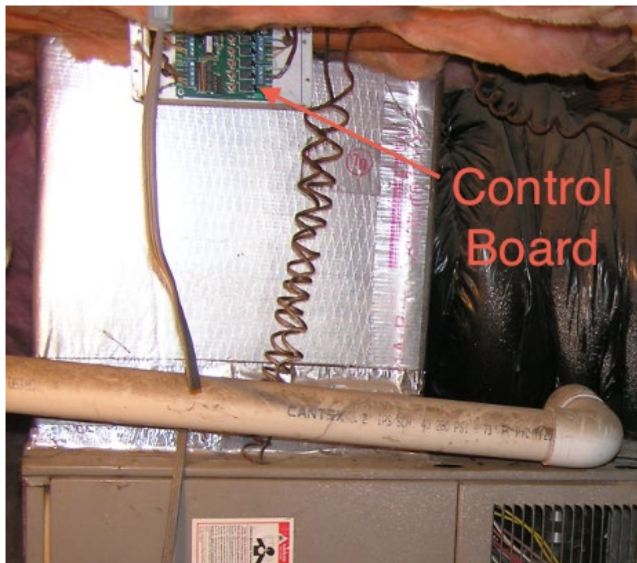
Figure C-6: Photo of a Duct-Mounted Control Board
