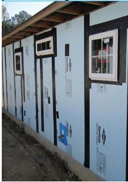
Figure 3-9: Properly Installed Rigid Insulation With Sealant Tape
