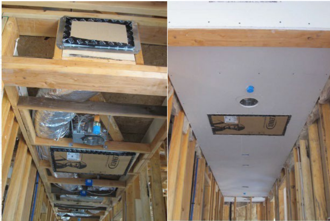
Figure 4-7: Ducts Routed Through a Dropped Ceiling
