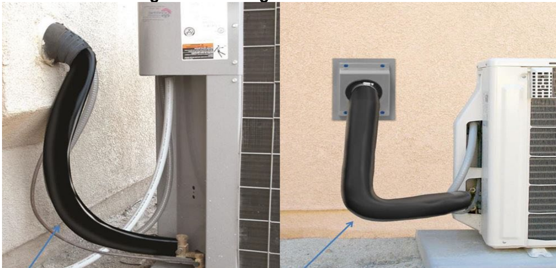
Figure 4-1: Refrigerant Line Insulation
