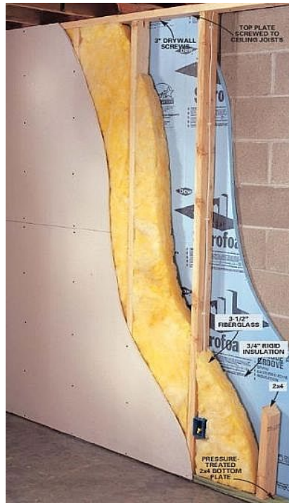
Figure 3-6: Brick Wall With Furring Details
