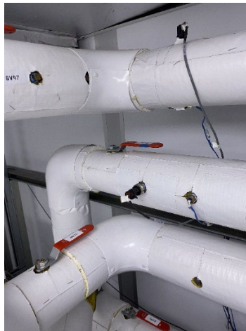
Figure 5-7: Continuous Pipe Insulation
