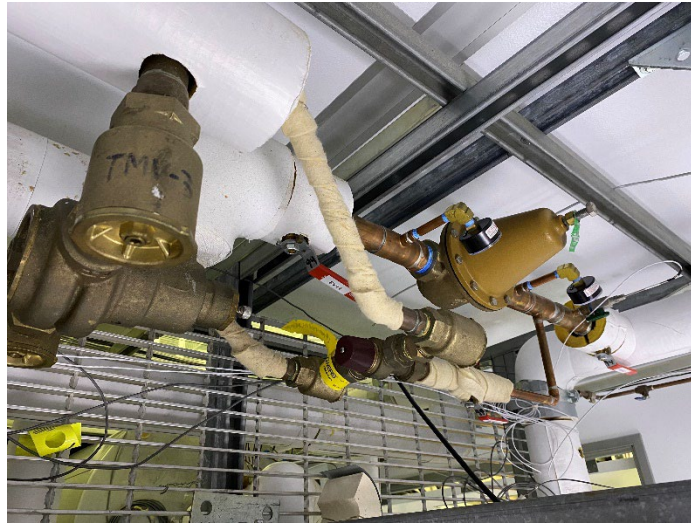
Figure 5-13: Image of a Two-Valve High Low Combination Thermostatic Mixing Valve
