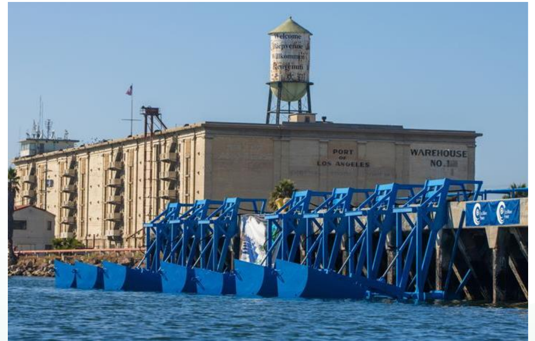
Eco Wave Power's wave energy converters installed at the Port of Los Angeles
