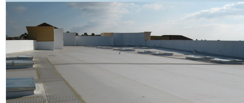
Cool roof coating at Palladio at Broadstone
