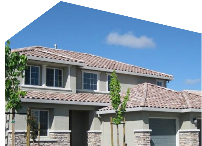
Tile roof on single family home.
