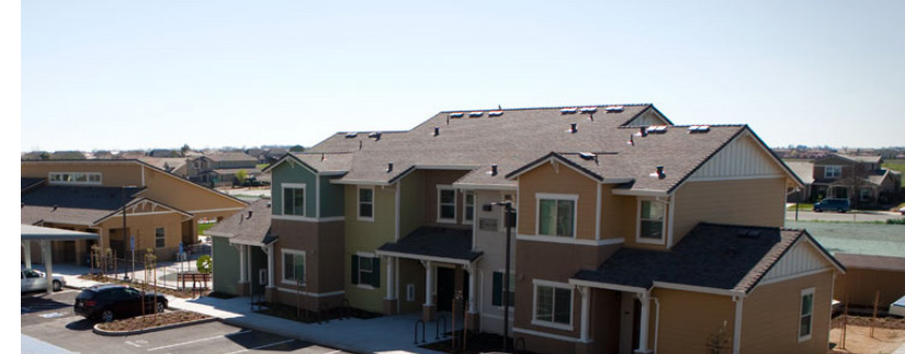
Asphalt shingle cool roof at Mutual Housing at Spring Lake.
