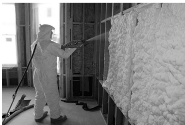
Figure 3-17: Open-Cell SPF Installed in Wall Cavity
