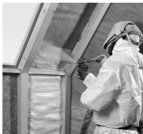
Figure 3-18: Closed-Cell SPF Installation in a Wall Cavity
