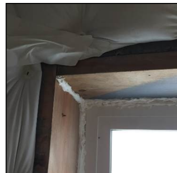
Figure 3-10: Air Sealing
