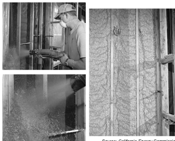
Figure 3-15: Cellulose-Insulated Wall
