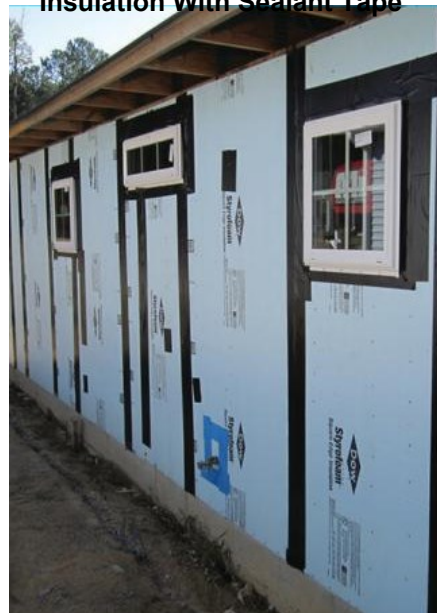
Figure 3-19: Properly Installed Rigid Insulation With Sealant Tape
