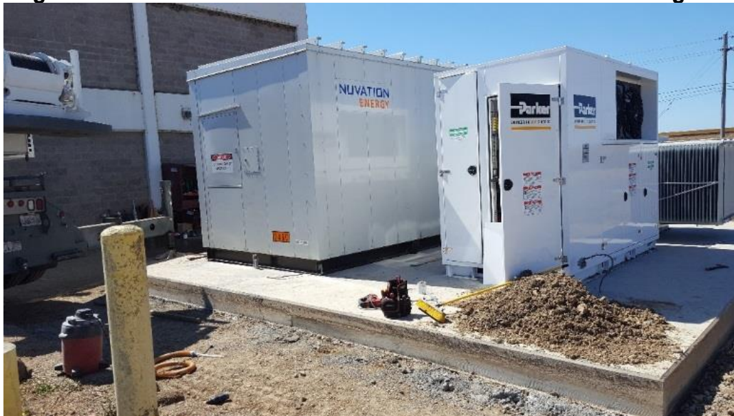
Figure 26: BESS Set In-Place and Electrical Connections In Progress
