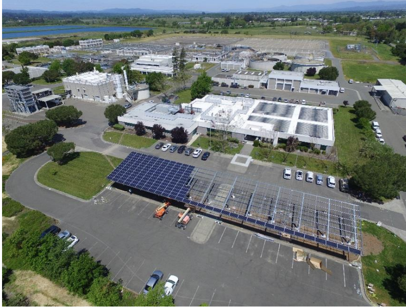
Figure 21: Contractor Begins Panel Installation at Carport Photovoltaic System
