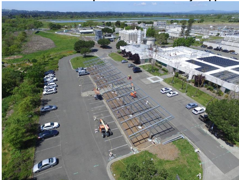
Figure 20: Aerial View of Carport Photovoltaic Array Support Structure
