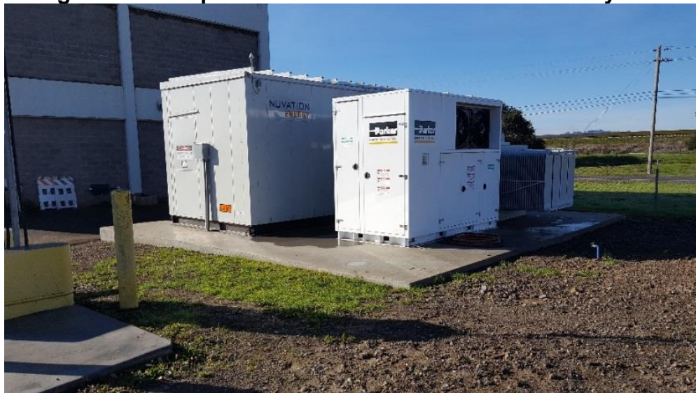
Figure 30: Completed BESS and Power Conversion System
