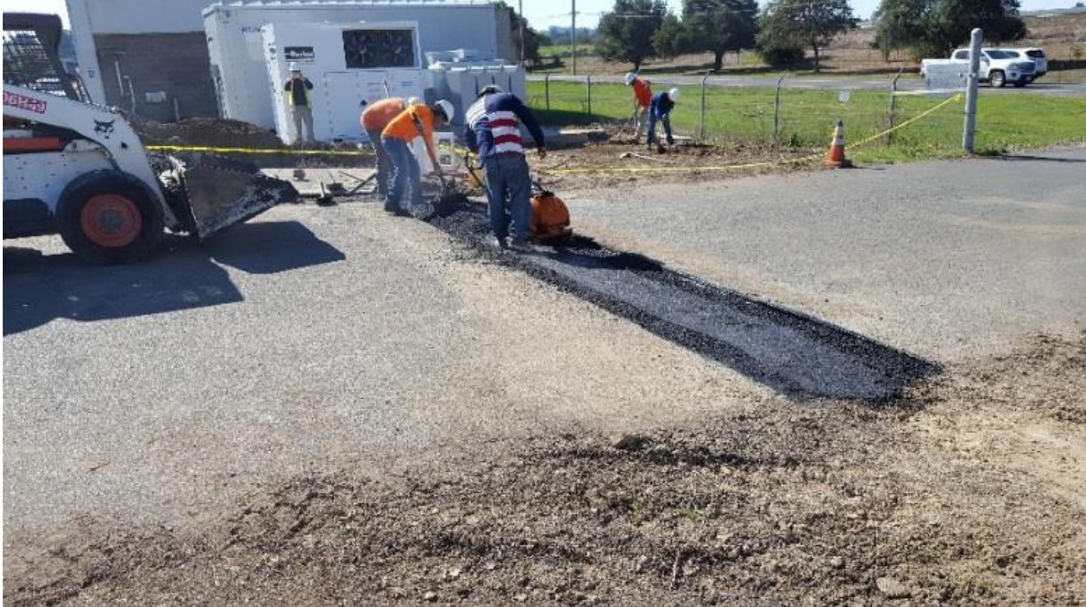
Figure 28: Completion of 12 kV Underground Installation to M2 Switchgear Tie-in
