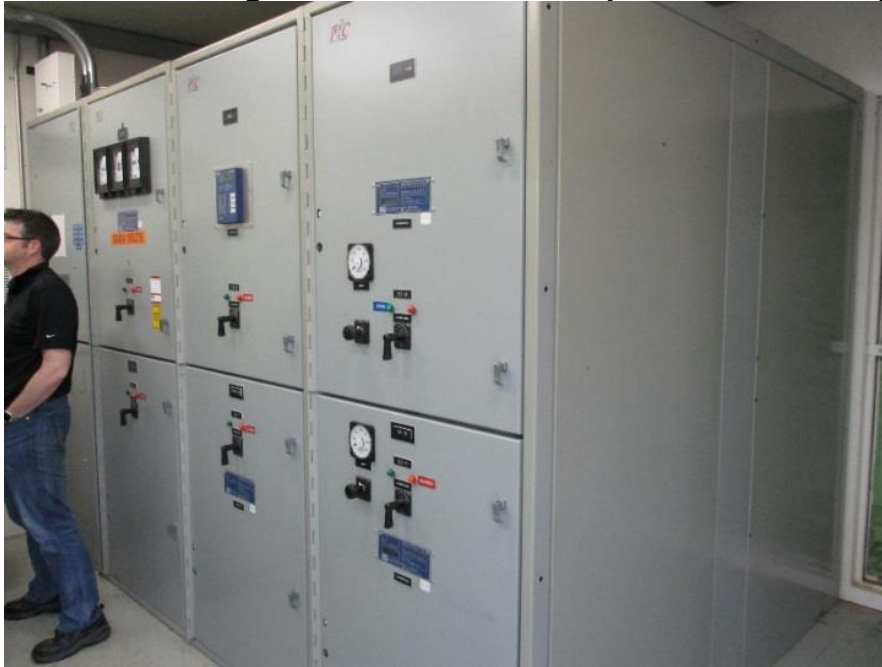
Figure 31: M2 Switchgear Modifications Completed for BESS System
