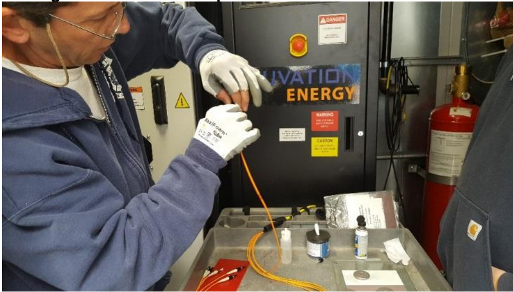
Figure 29: Final Fiber Optics Communication Connections
