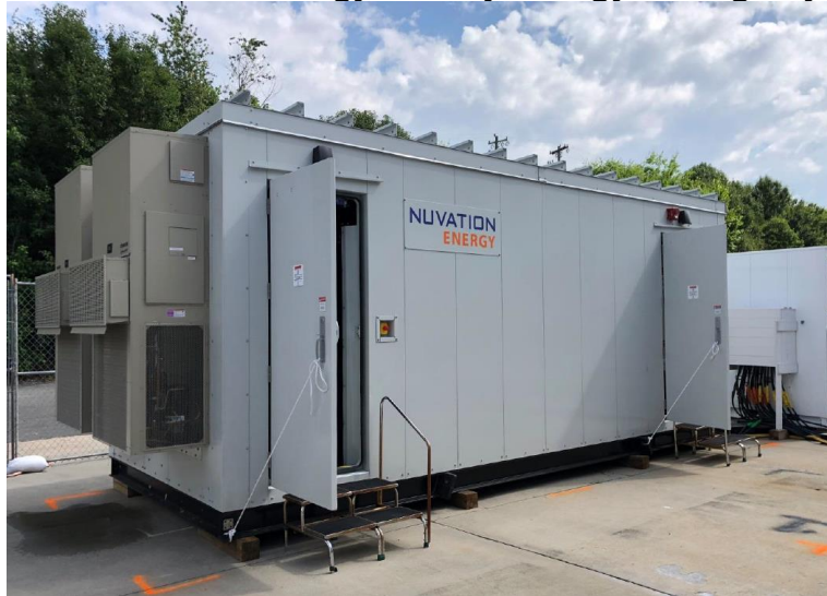
Figure 8: Nuvation Energy Battery Energy Storage System
