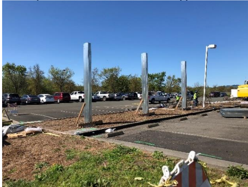
Figure 19: Carport Photovoltaic Structural Support Post Installation
