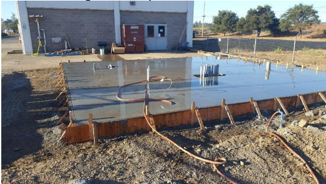
Figure 25: Completed BESS Pad Area
