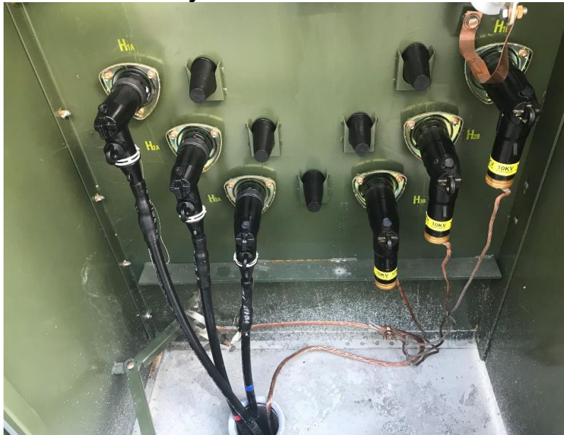
Figure 27: Power Conversion System Transformer Final Connections Completed
