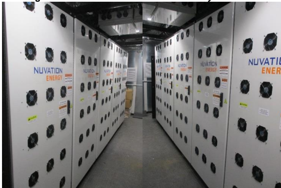
Figure 33: Inside View of the BESS Battery Container
