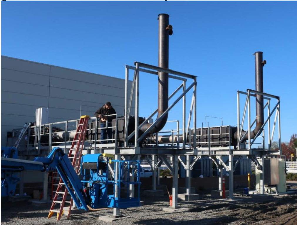
Figure 7: Two Miratech Selective Catalytic Reduction Unit Installations
