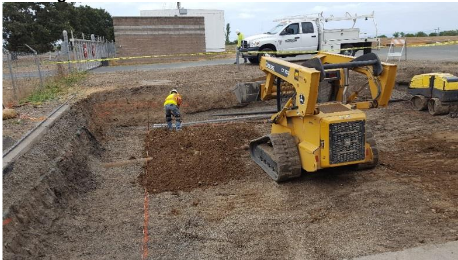
Figure 23: Excavation of BESS Concrete Pad Area
