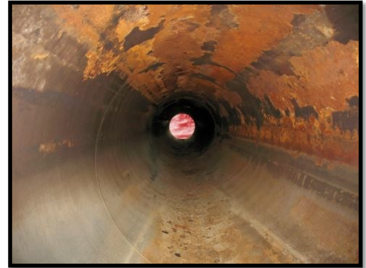
Photograph of internal corrosion in pipelines. Source: https://cdn.corrosionpedia.com/images/uploads/tunnel.jpg?height=580&width=940
