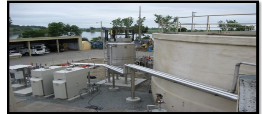
Photograph of microturbines, gas cleanup system, and digester. Source: Las Gallinas Valley Sanitary District
