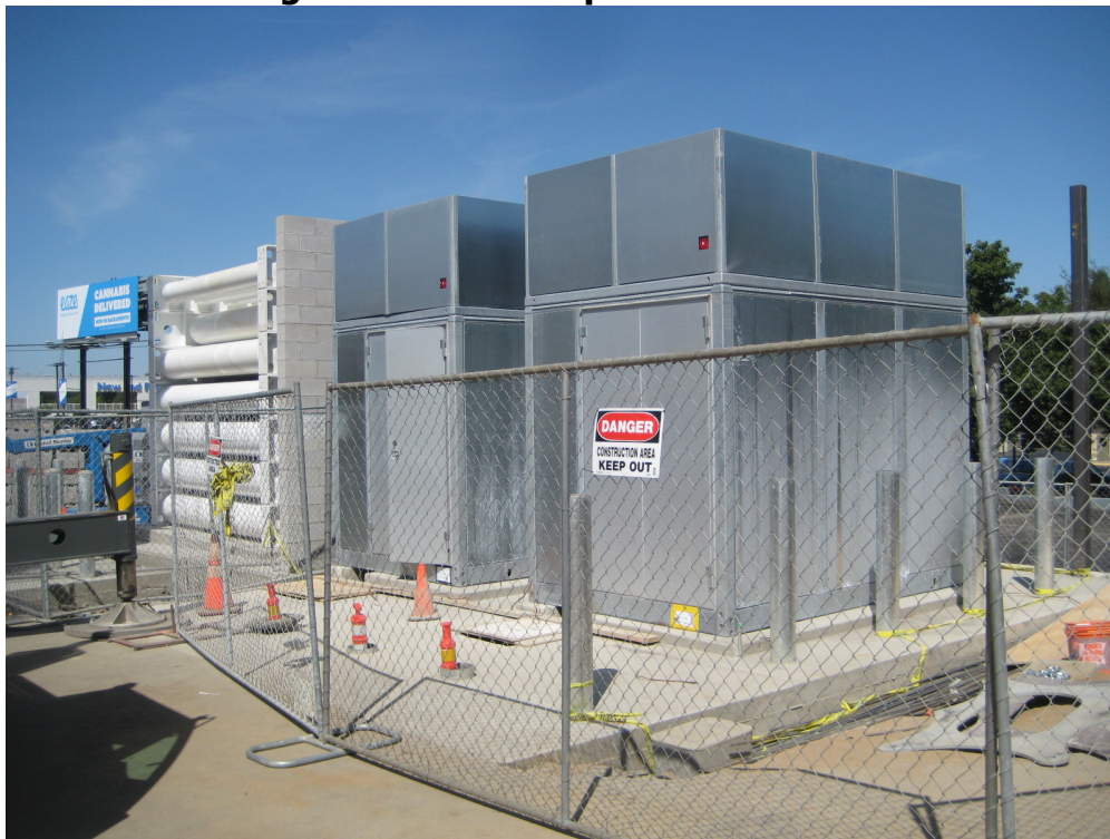
Figure 5: Two Compressor Modules
