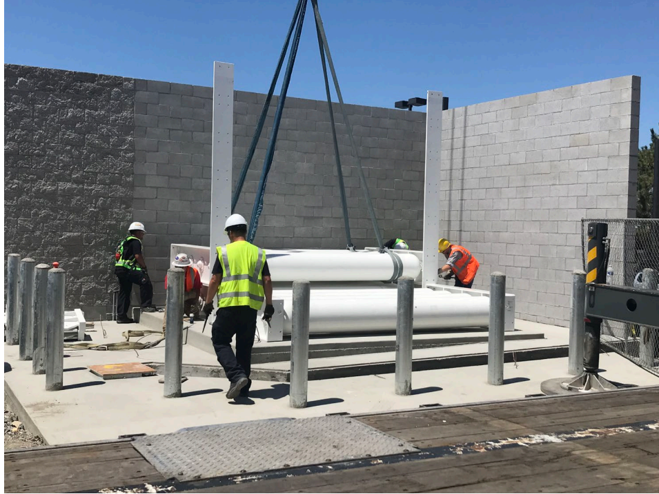
Figure 4: Field Assembly of Storage Module
