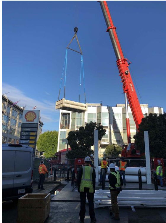
Figure 4: Field Assembly of Storage Module
