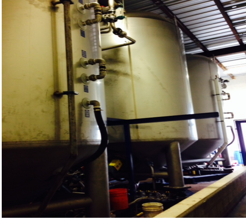
Figure 6: All Three Reactors in Place and Piped in
