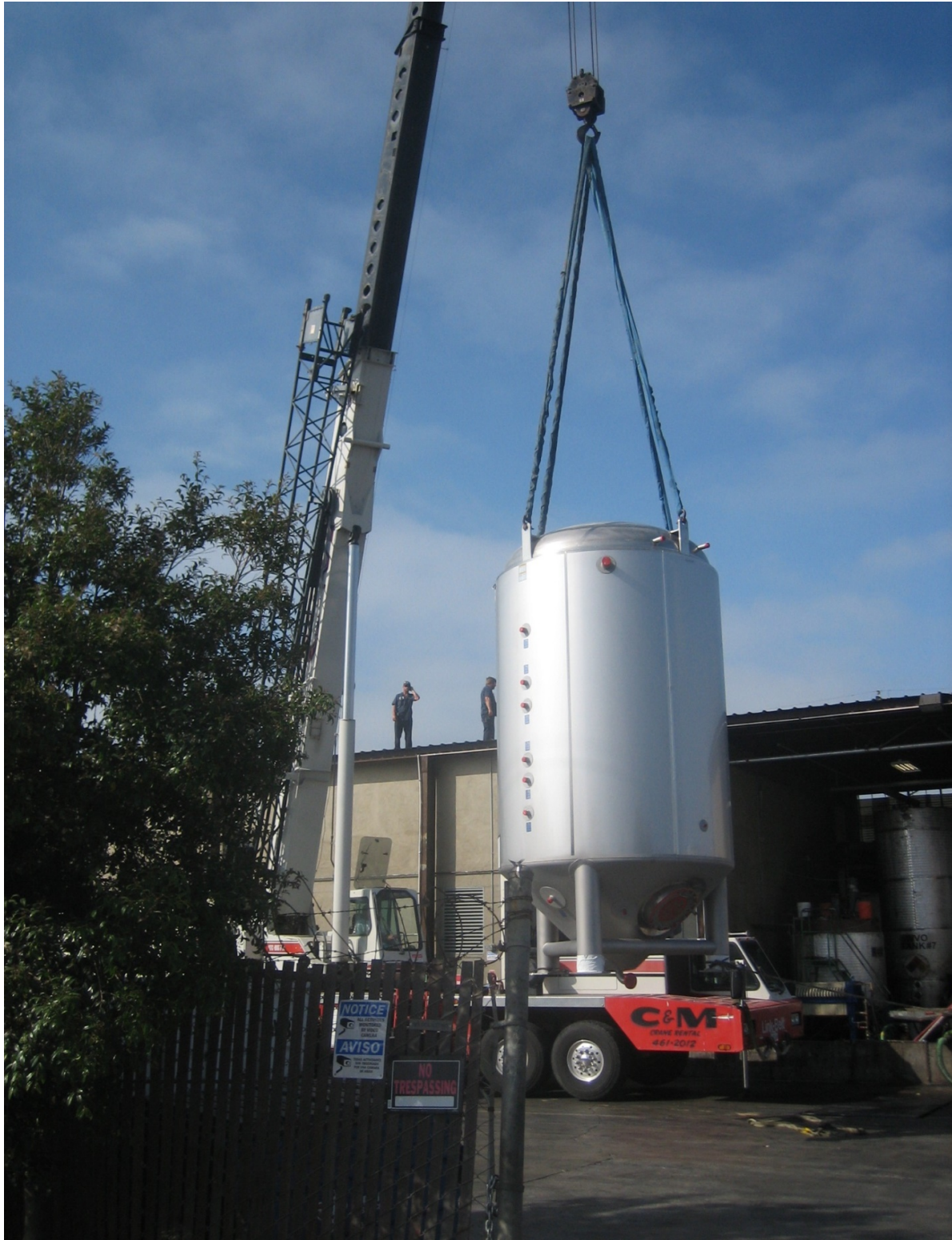
Figure 4: Tanks Hoisted into Processing Room Through Roof
