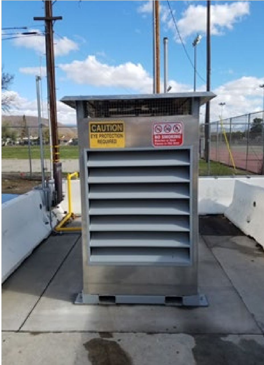
Figure 5: Compressor Housing at Lindsay Unified School District Transportation Yard
