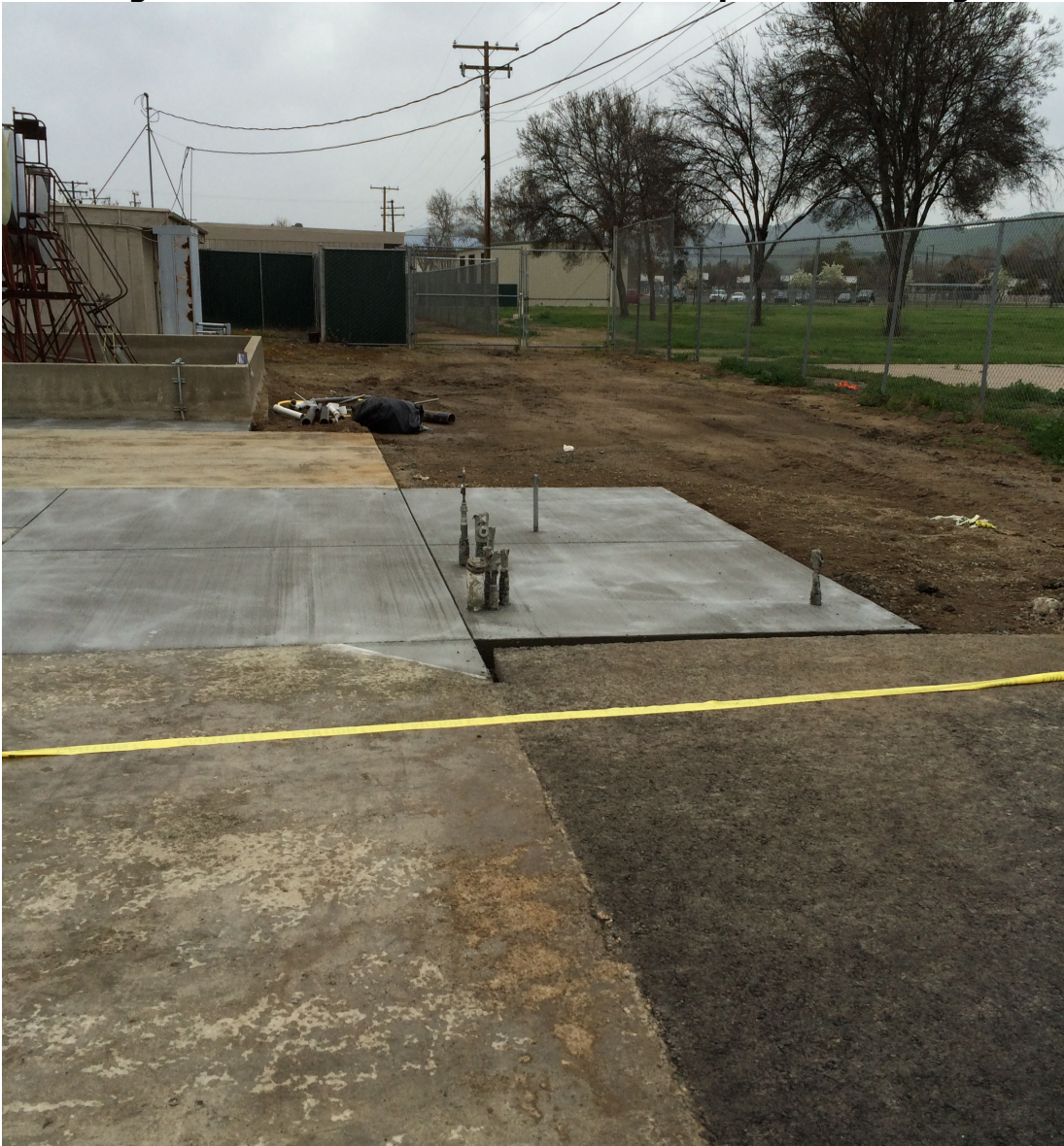
Figure 6: Concrete Slab Poured for Compressor Housing
