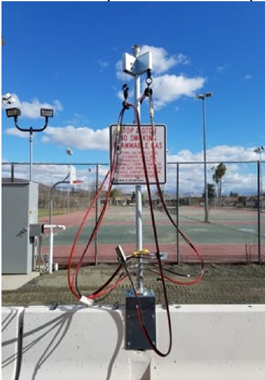
Figure 4: Time-Fill Post at Lindsay Unified School District Transportation Yard
