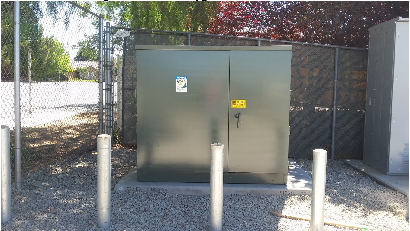
Figure 4: Electrical Upgrades for CNG Station
