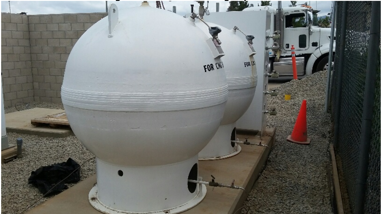
Figure 3: Relocated Storage Spheres
