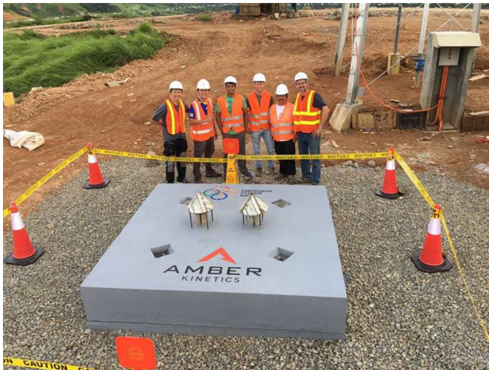
Figure 12: Demo Installation at Subic Bay, Philippines
