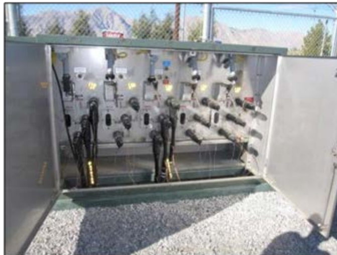
Figure 9: Five-Way Underground Switch
