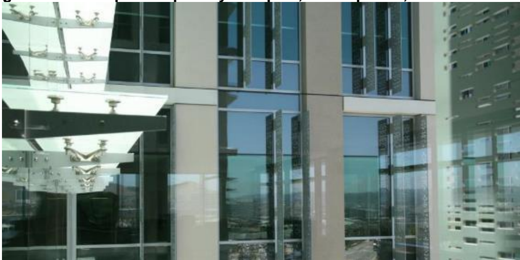
Figure 5.1: Example of Optically Complex, Noncoplanar, Exterior Shading
