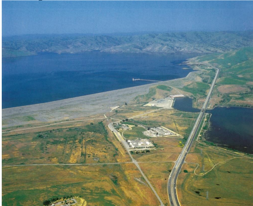
Figure 7: Aerial View of San Luis Reservoir
