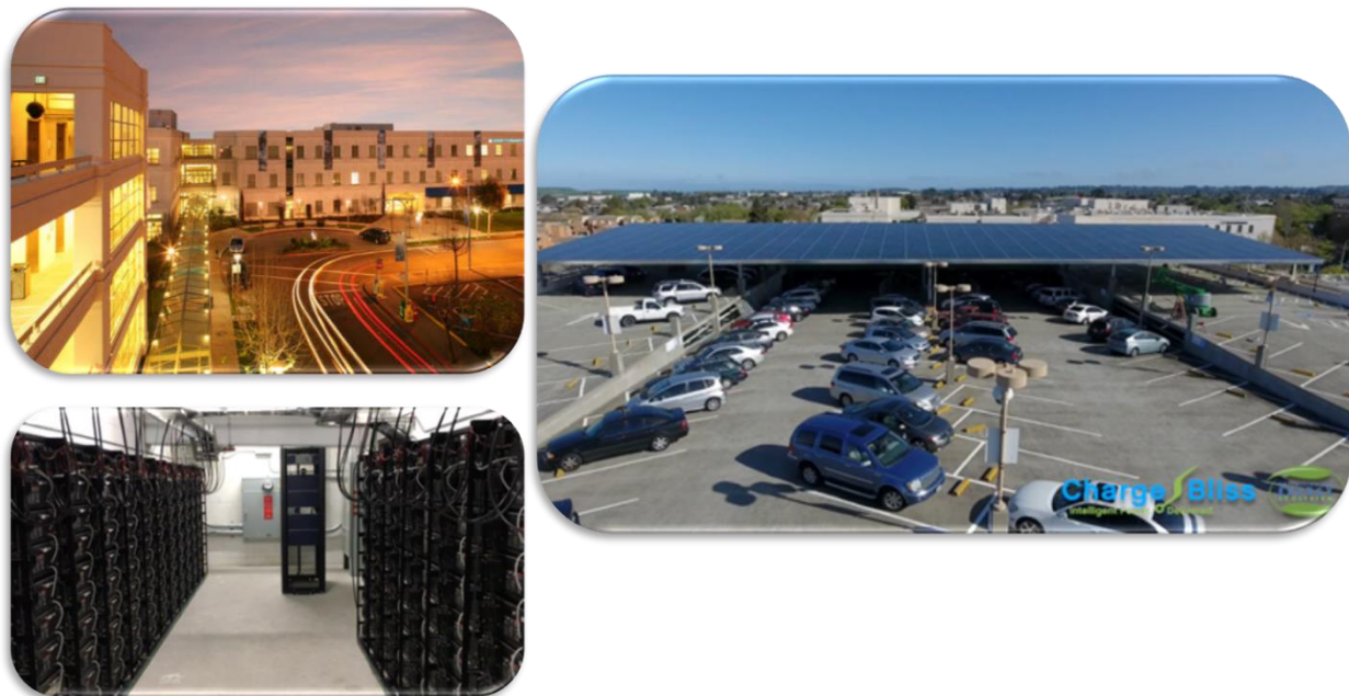
Figure 10: A Renewable Energy Microgrid for Kaiser Richmond Medical Center
