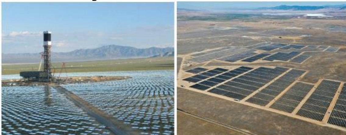
*Left:* The 392 MW CSP Ivanpah Solar Thermal power plant. *Right:* The 250 MW tracking PV California Valley Solar Ranch (CVSR) power plant.
