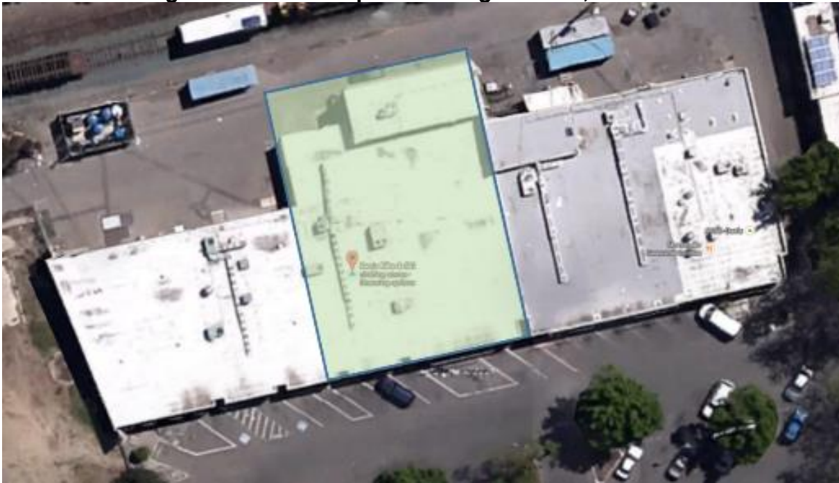
Figure 86: Aerial Map of Building in Davis, California
