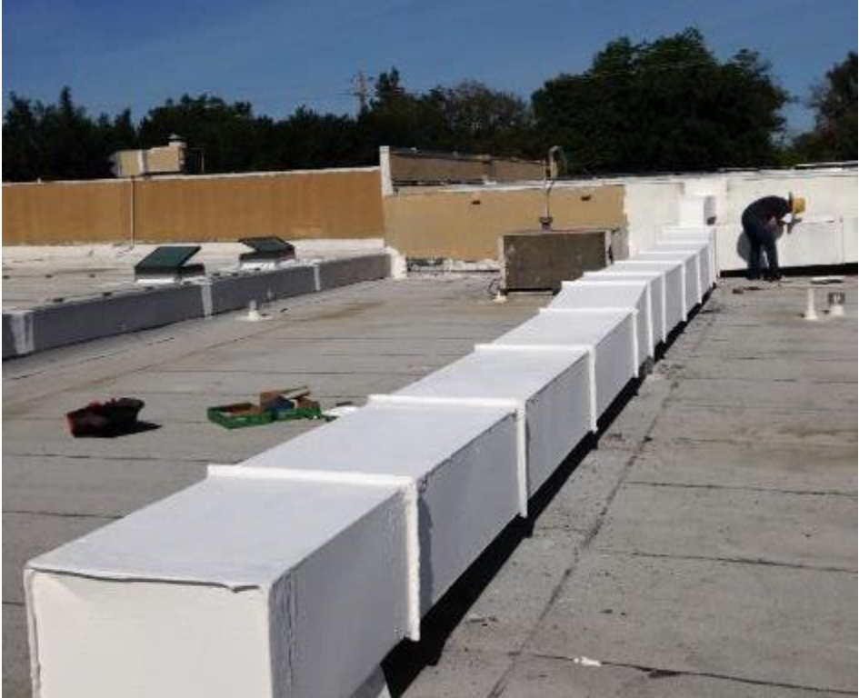
Figure 94: Post-Retrofit of Exposed Supply Ductwork at Dry Cleaning Tenant
