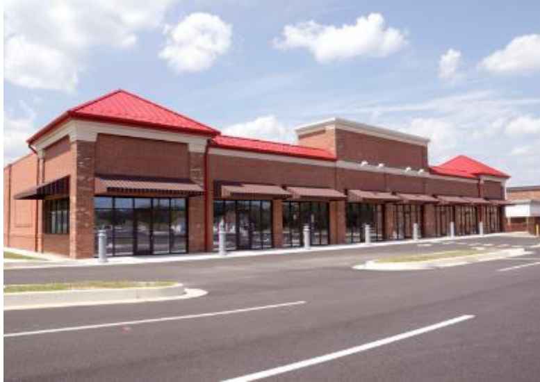
Figure 35: Multitenant Light Commercial Building with Window Awnings
