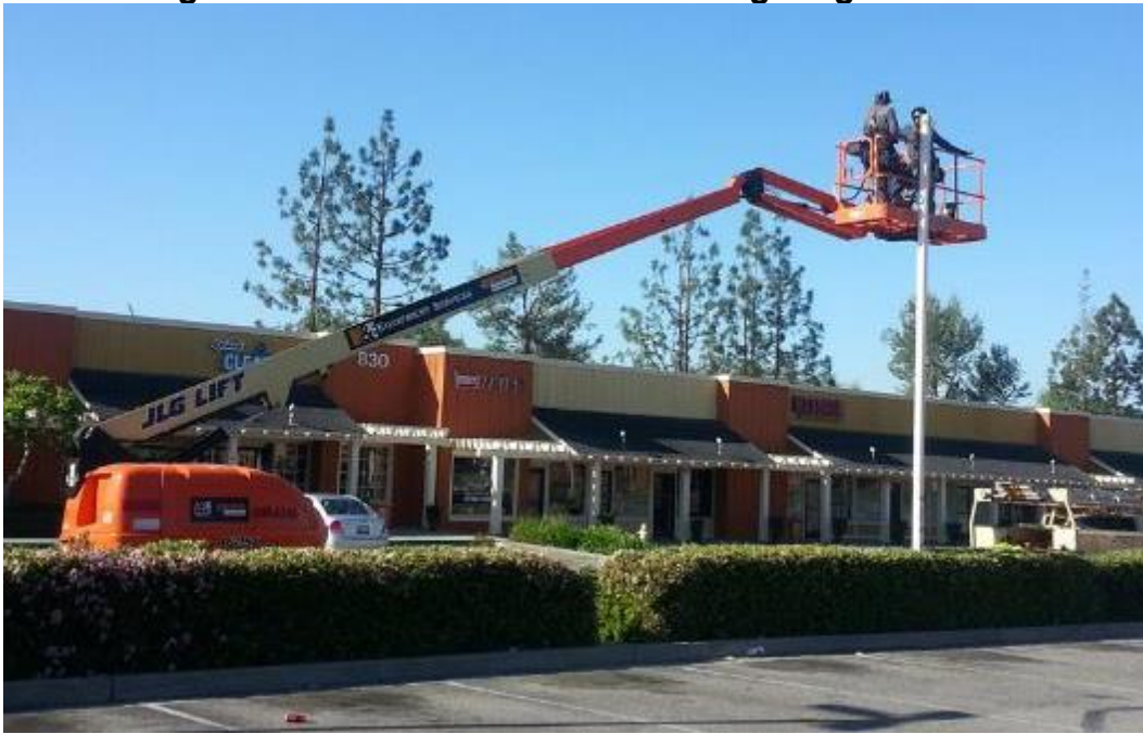
Figure 106: Installation of the LED Lighting Measure
