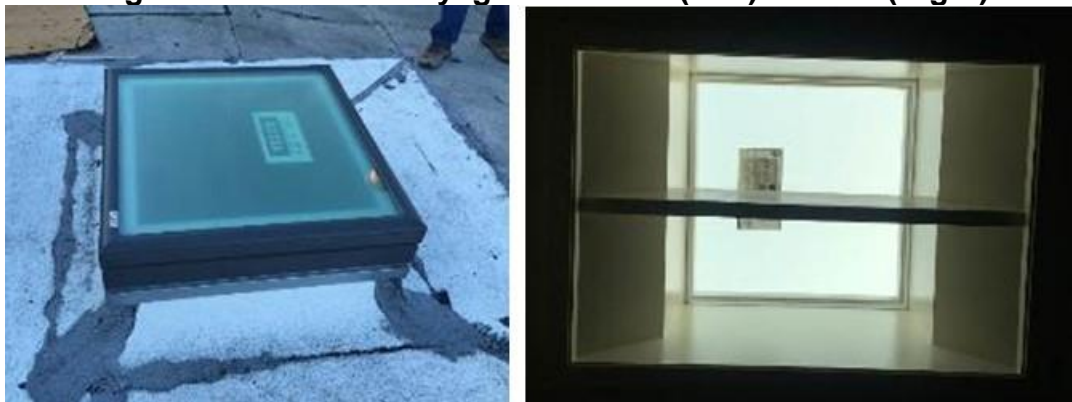
Figure 90: Finished Skylights Exterior (Left) Interior (Right)
