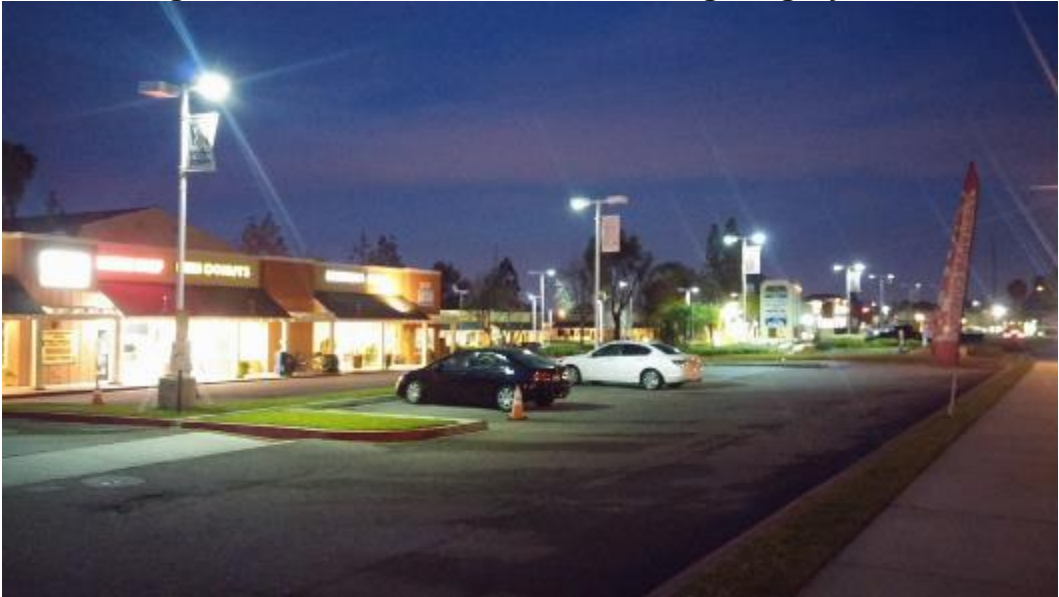
Figure 105: Pre-Retrofit of Exterior Lighting System
