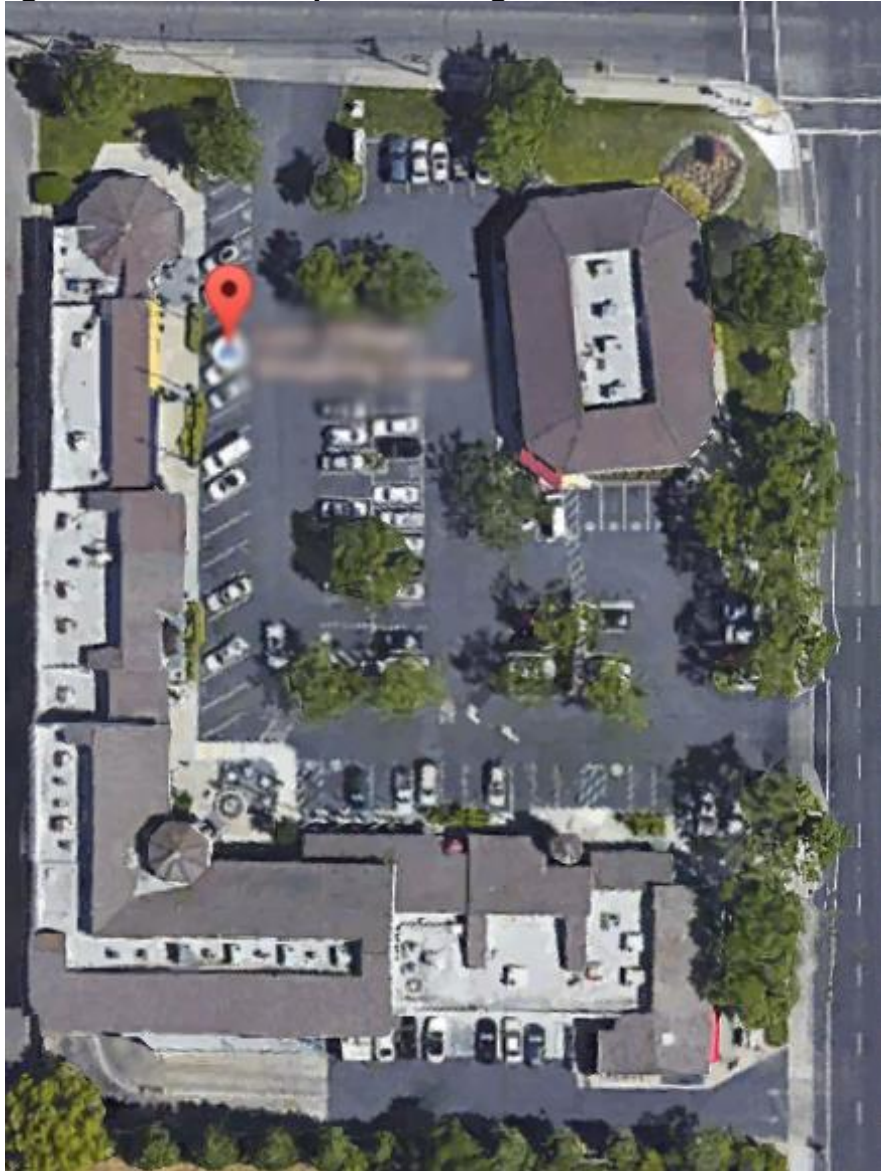
Figure 108: Aerial Map of Building in Sacramento, California
