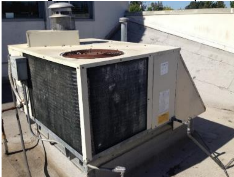
Figure 110: Pre-Retrofit of Rooftop
