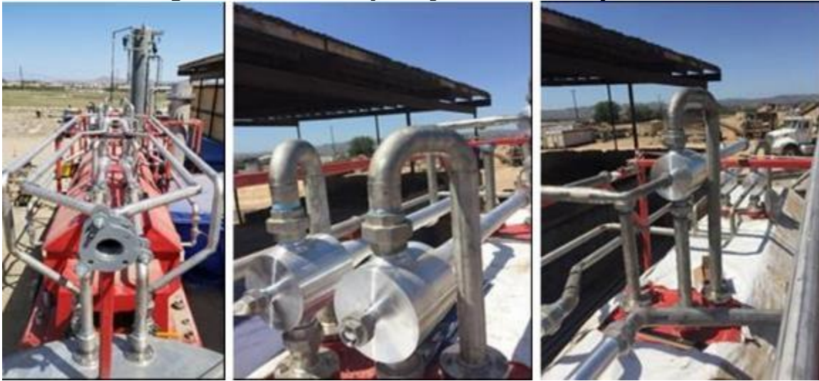
Figure 22: Assembly of Ejector-Based System
