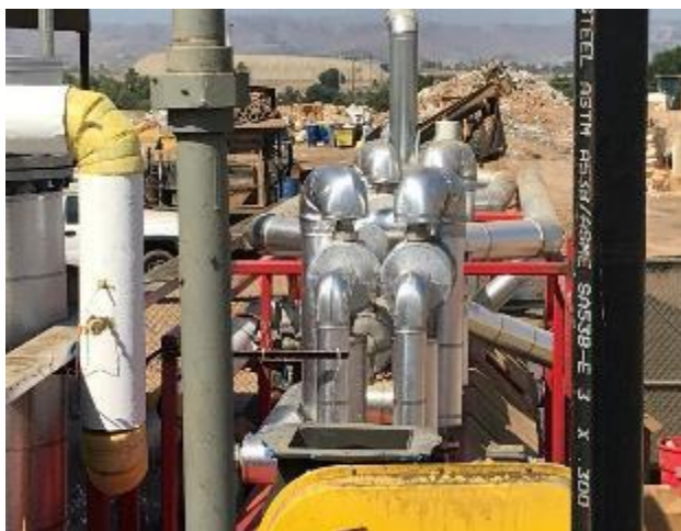
The ejector-system was steam pressurized and thermally insulated
