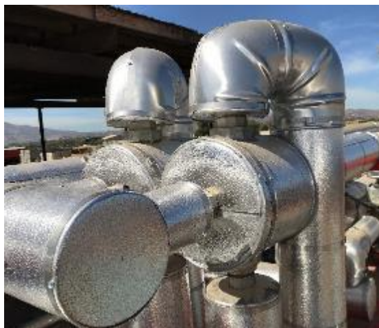
The ejector-system was steam pressurized and thermally insulated
