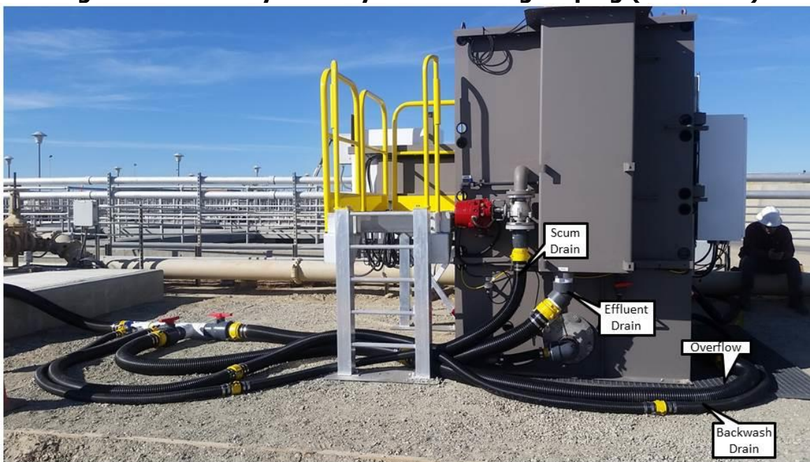
Figure 21: Primary Filter System Discharge Piping (Lancaster)
