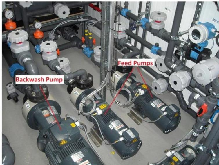
**Figure 2-5** Photo of Pilot Unit Pumps
