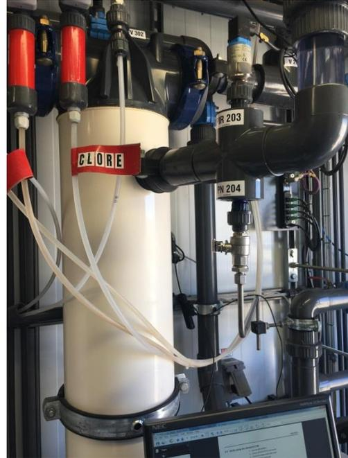
**Figure 2-4** Photo of Standard UF Membrane
