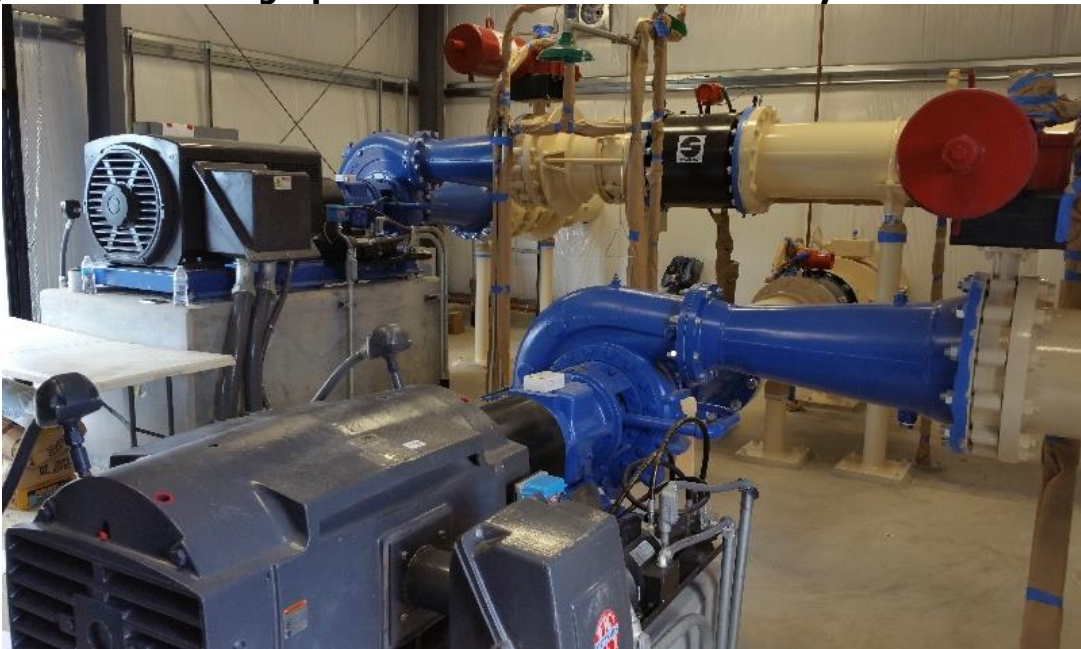
Figure A-35: Photograph of the PAT Units in Perdue Hydroelectric Station
