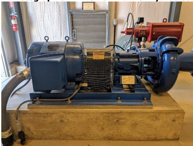
Figure A-7: Photograph of PAT Unit in Tanner Hydroelectric Station
