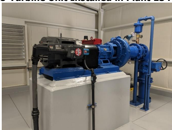
Figure A-13: Pump-as-Turbine Unit Installed in Plant 134 Hydroelectric Station
