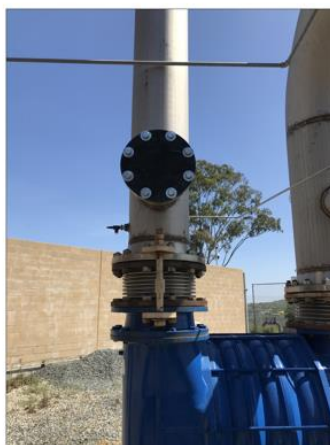
Feed to compressor trailer capped off
